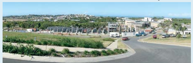
Seaspray units Stage 1 is the design and construction of 17 open plan two and three-bedroom luxury units.
